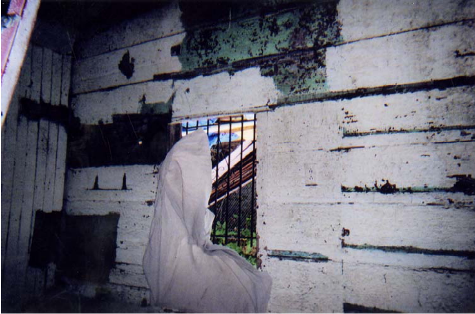
Figure Five The home in 2005 before the renovation
